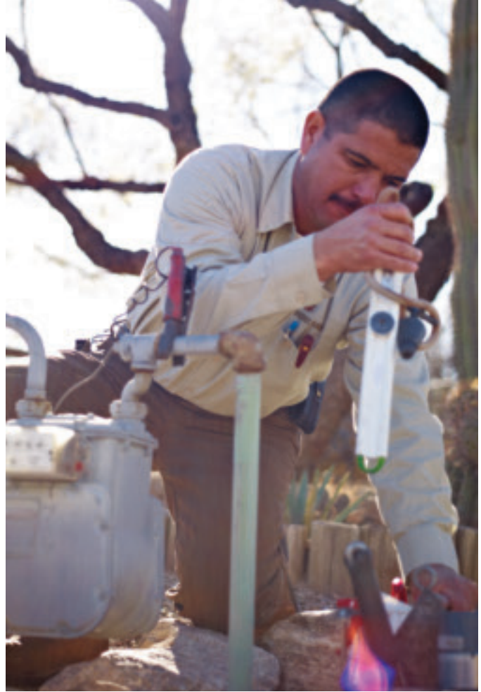
Manny Corral works to replace a COYL in southern Arizona.
